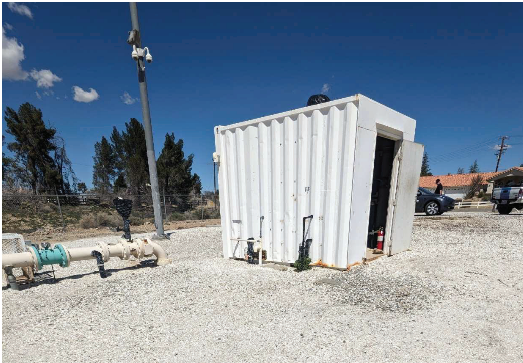
Figure 3. Disinfection Equipment Container for Well 18.
