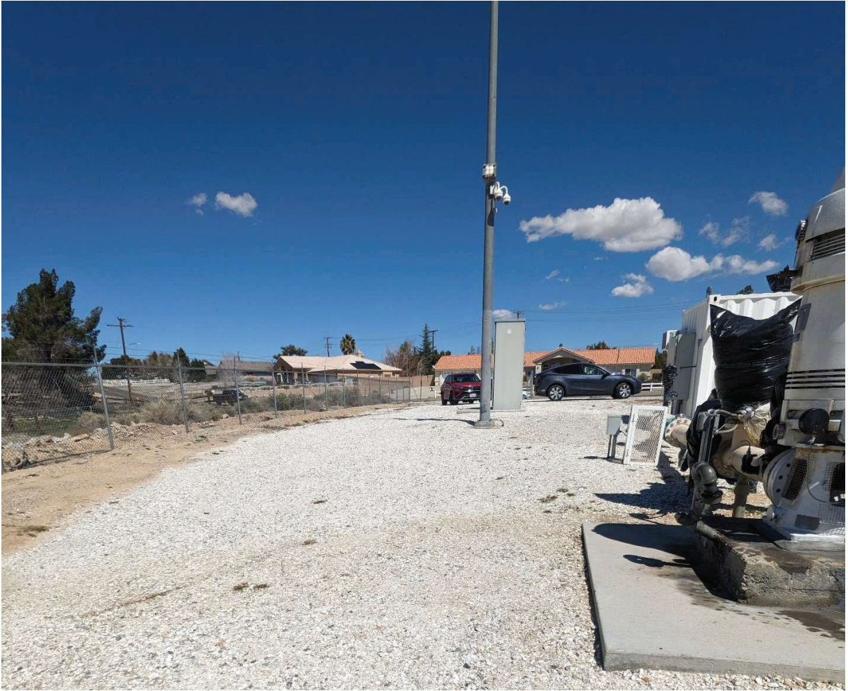
Figure 4. View of Well 18 lot.
