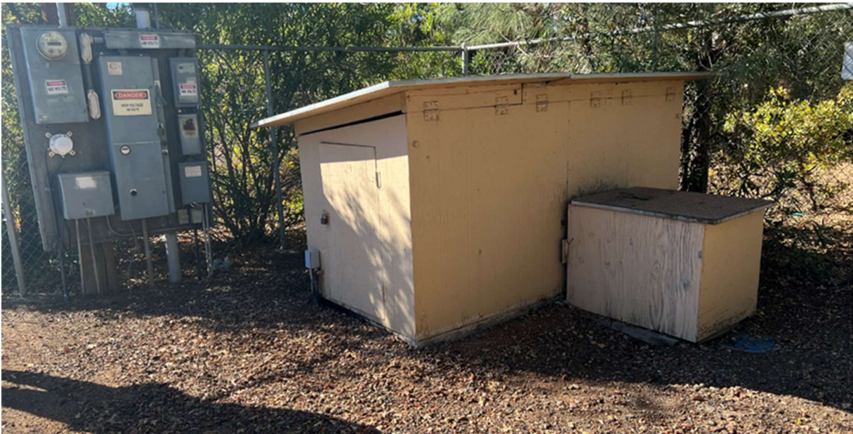
Figure 3-1. Cal Advocates field trip to Manchester plant site on October 30, 2023
